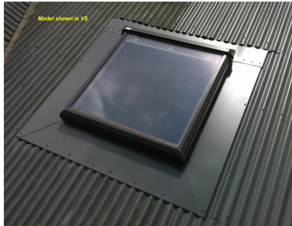
Purpose-built flashing with top tray under roofing material
